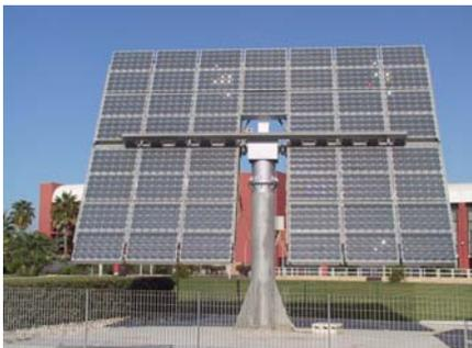
Fig. 1. The 5kW<sub>p</sub> PhoCUS standard unit
